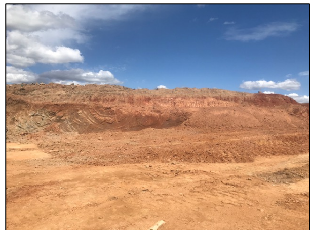
Earthworks undertaken in southern area of site
